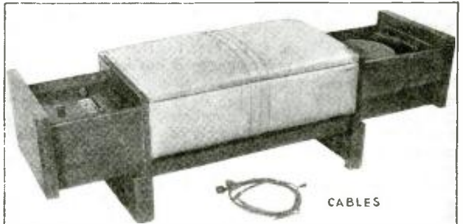
This is the piano-bench of the "Storytone". The modern radio set in one sliding drawer, and the electric phonograph in the other, are optional.
